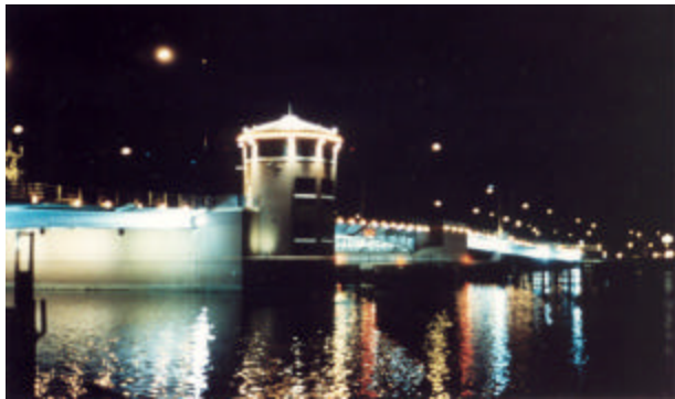
US Lamp was instrumental in the lighting of Green Bay's Ray Nischke Memorial Bridge
